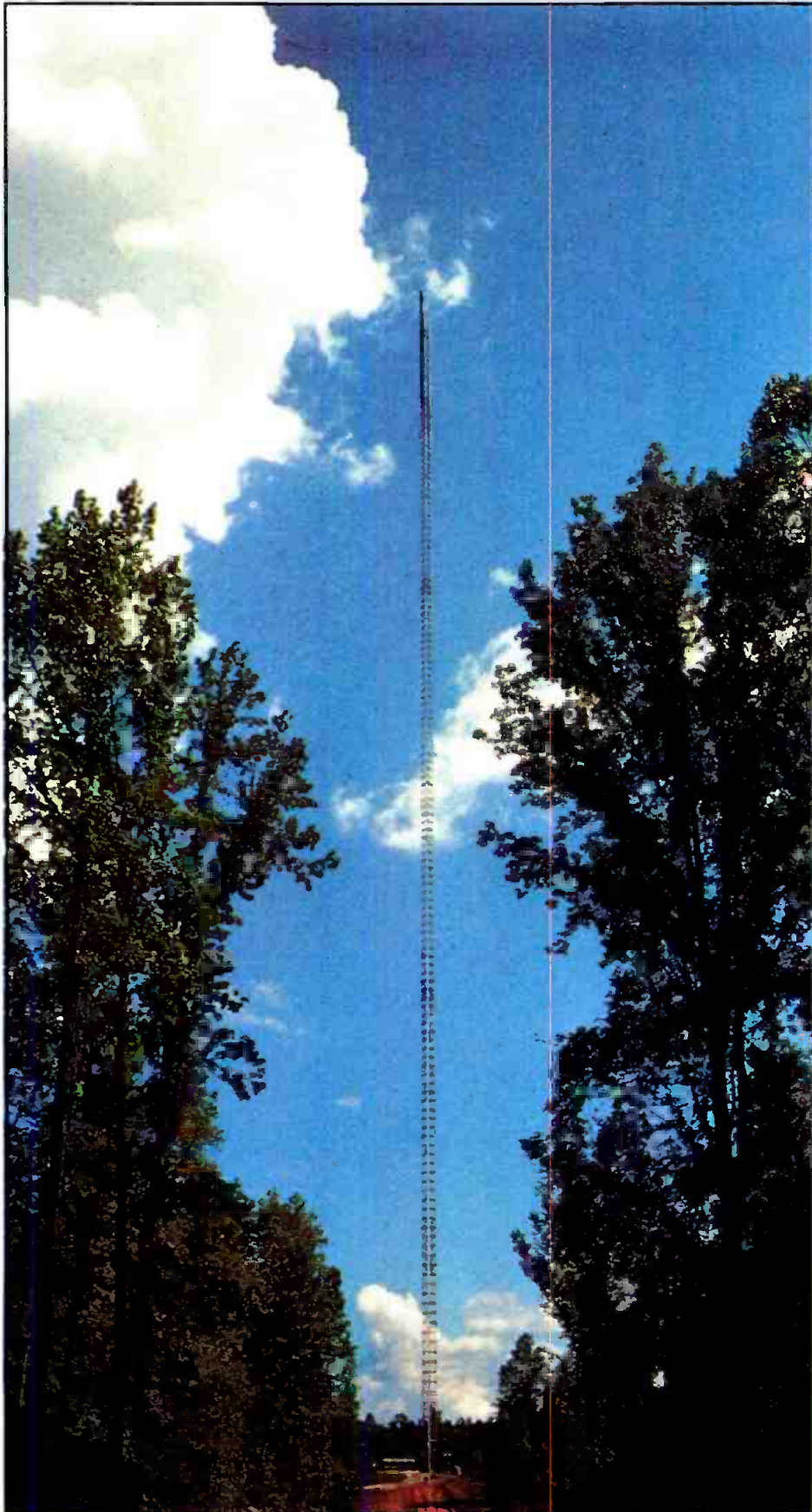
The 1764-foot transmitting tower of WFOX-FM, Atlanta, GA.
